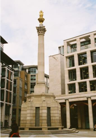
“Cunningly disguised ventilation shaft”
