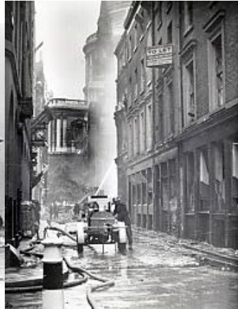
QUEEN VICTORIA STREET (No.25), collapsing in flames, as a result of incendiary bombs, dropped during an air raid 10th - 11th May, 1941.
